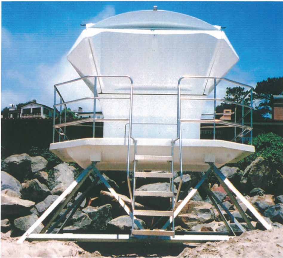
APEX lifeguard tower left and bottom photos, shutters are down and latched, securing the tower.
