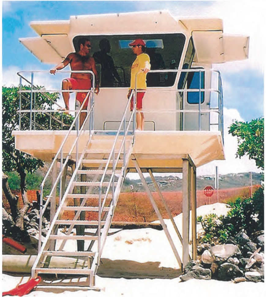
Sandy Beach Park, Oahu, Hawaii Permanent site stainless steel structure, 35 degree low angle stairs.
